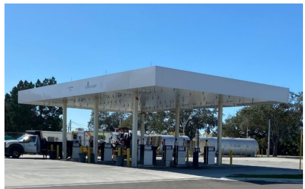
Breeze Diesel Fueling Station Source: Benesch
