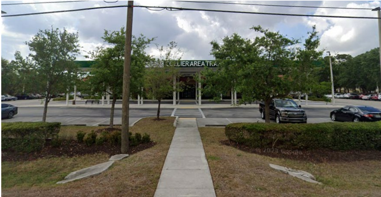
Figure 2-3: CAT Radio Road Transit Facility (Source: Google Street View)
