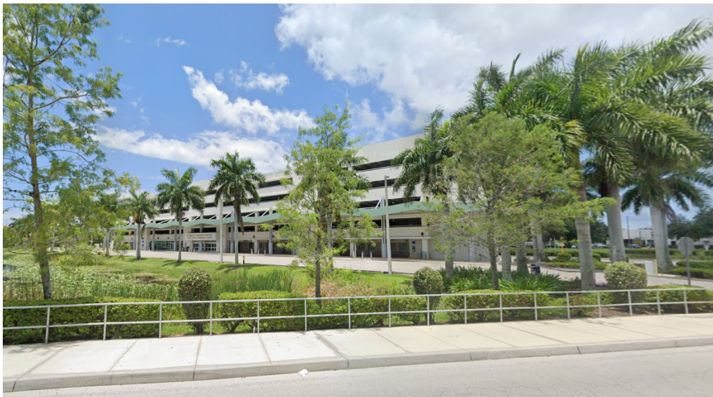
Figure 2-4: Intermodal Transfer Station (Source: Google Street View)
