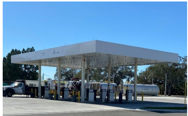
Breeze Diesel Fueling Station Source: Benesch
