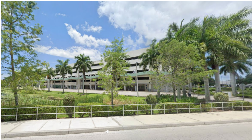
Figure 2-5: Intermodal Transfer Station (Source: Google Street View)
